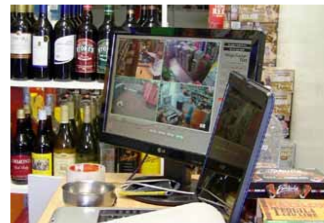
EXAMPLE OF CCTV MONITOR
