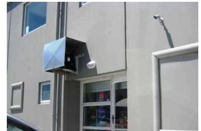
EXAMPLE OF CCTV AT REAR OF PREMISES
